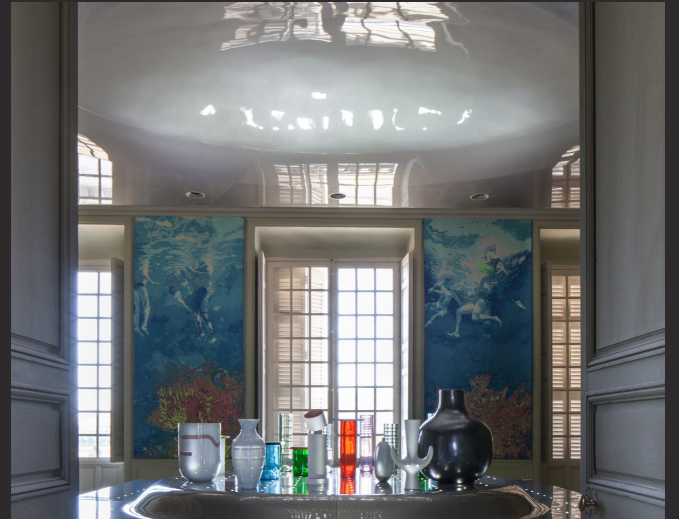
Lacquered ceilings in composite materials for the BORELY Museum of Decorative Arts by the MOATTI and RIVIERE Architectural Agency.
